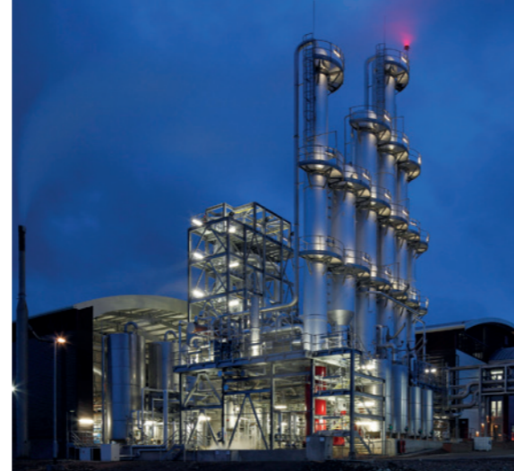
Glen Turner, Scotland - complete distillery for 75,000 l/day Whisky and alcohol production
